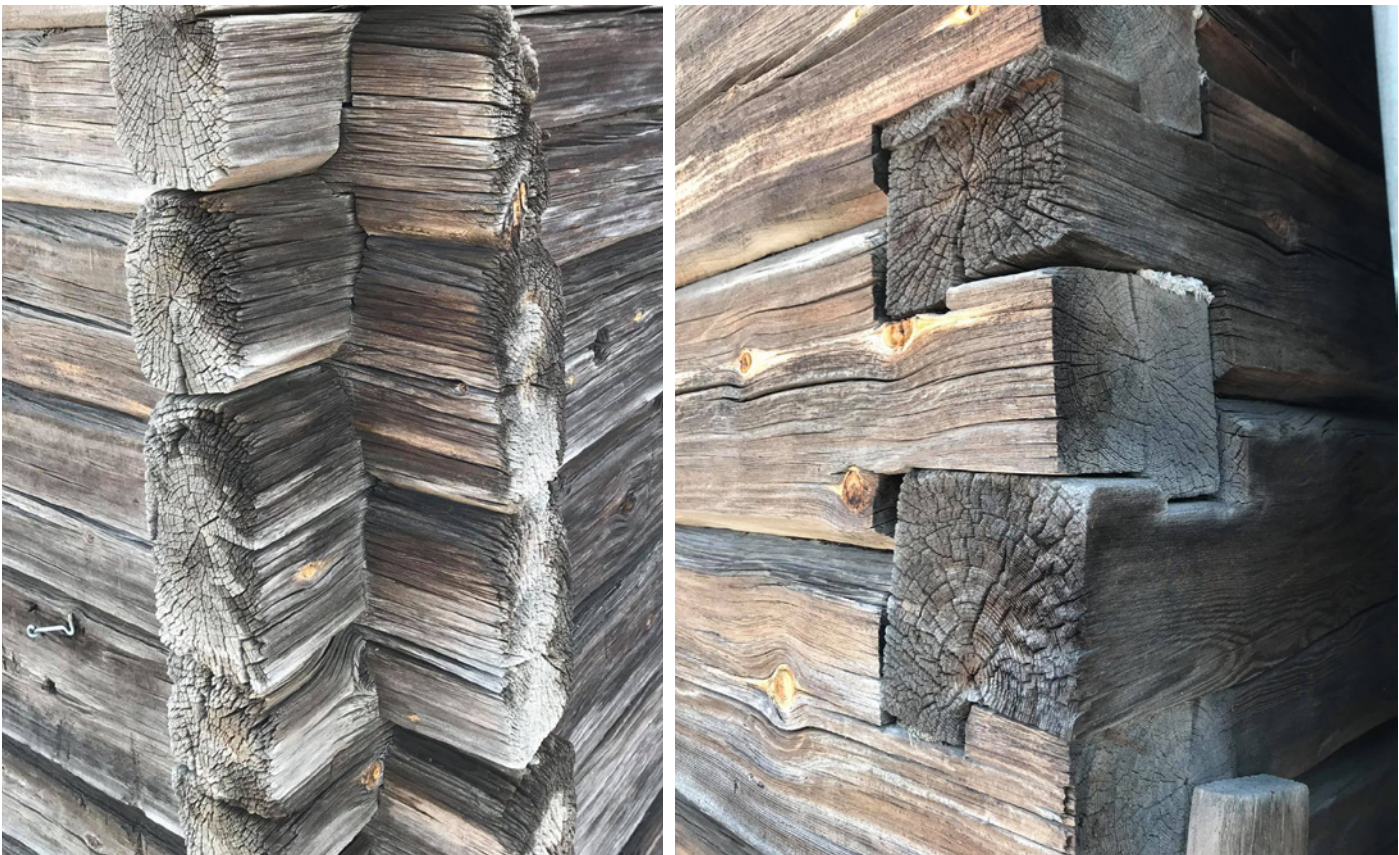
Picture 11. Two common corner joints found in the church village of Öjebyn, Piteå, source: authors
